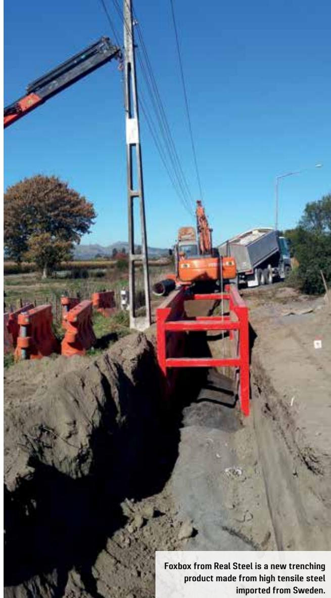
Foxbox from Real Steel is a new trenching product made from high tensile steel imported from Sweden.
