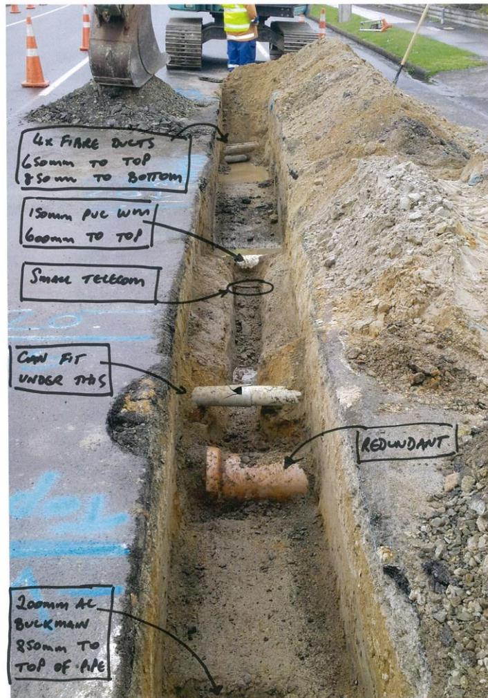
**Photo 2: Services in the path of proposed stormwater pipeline**
