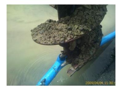
Reference: OT011 Material: PE Description: Pipe strike. Cause: Third party. Repair; Replace damaged pipe.
