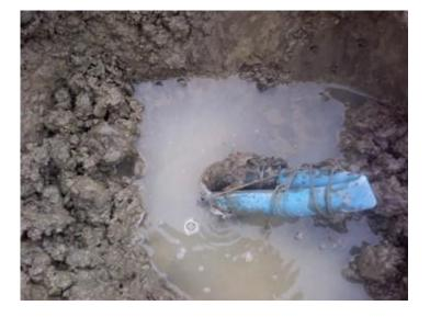
Reference: EX006 Material: PE Description: Emergency seal Cause: Pipe folded back to provide emergency seal. Comment: Temporary repair method.
