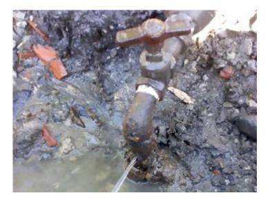
Reference: EX004 Material: Copper Description: Corroded pipe Cause: Shaking and corrosion. Repair: Replace damaged pipe.
