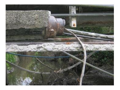
Reference: OT004 Material: Cast iron encased in concrete Description: Break
