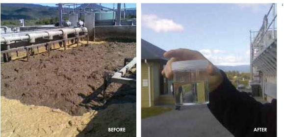
Figure 2 - Comparison of solids level in MBR tank and treated water
