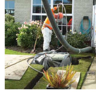
"The Stronger Christchurch Infrastructure Rebuild Team (SCIRT) is designing, managing and delivering the infrastructure rebuild. E/One pressure sewers were identified as a key technology to provide costeffective, permanent wastewater service to a number of catchments with significant damage to the gravity network or significant risk of damage from future seismic events."
