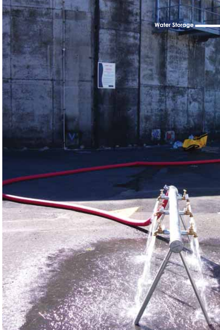
Figure 2 – Capacity Emergency Manifold Stand at Reservoir
