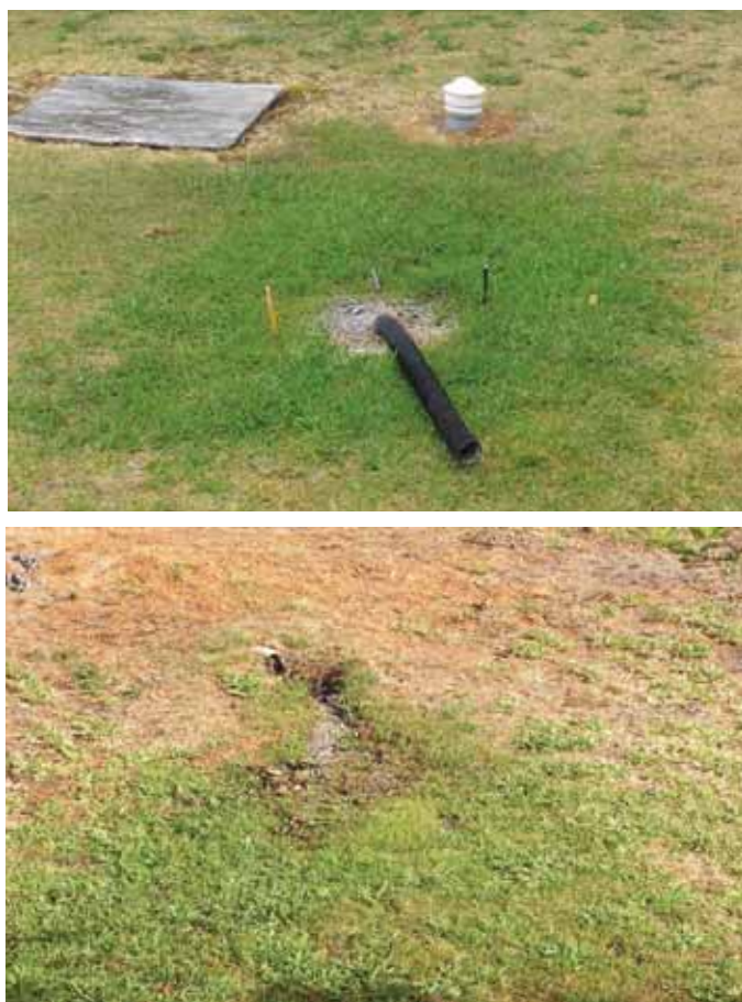
Figure 1 – Typical greywater outlets as found in the case study community on the west coast of North Island
