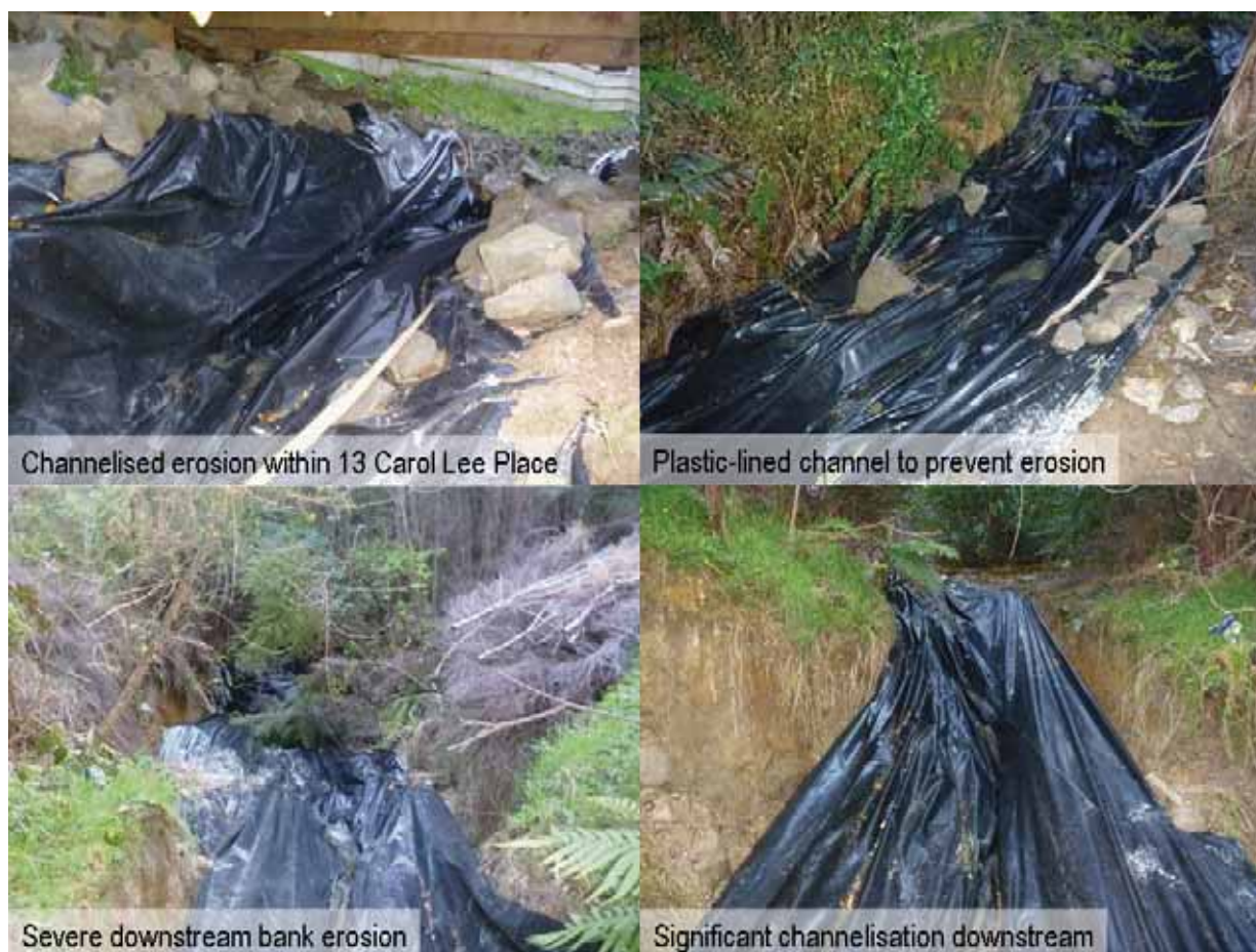
Figure 10 – photos taken during site visit on 9 September 2011, illustrating severe downstream erosion
