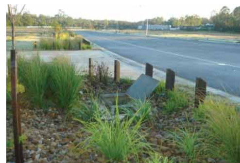
Bioretention basin at Arundel, Gold Coast, designed by OPUS
