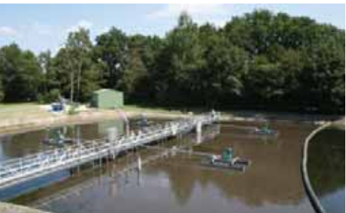
Figure 3 – CWSBR® System under running conditions, showing aerated zone
