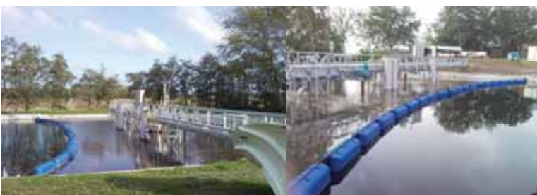
Figure 5 – CWSBR® Control Bridge and Hydrosail separating activated sludge zone from clear water zone
