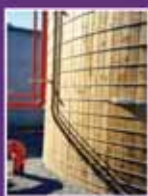
Fire Protection Tank
