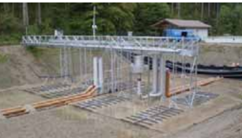
Figure 2 – CWSBR® is a full performance SBR process in the shape of a pond technology, which grants highest wastewater treatment standards
