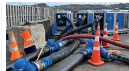
The Netherlands-designed pumps, overpumped 928 million litres of wastewater during the project.
