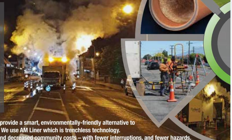
New Zealand owned and operated since 2003, we provide a smart, environmentally-friendly alternative to traditional small bore pipe rehabilitation methods. We use AM Liner which is trenchless technology. This means: no digging - so less time on the job, and decreased community costs – with fewer interruptions, and fewer hazards.
