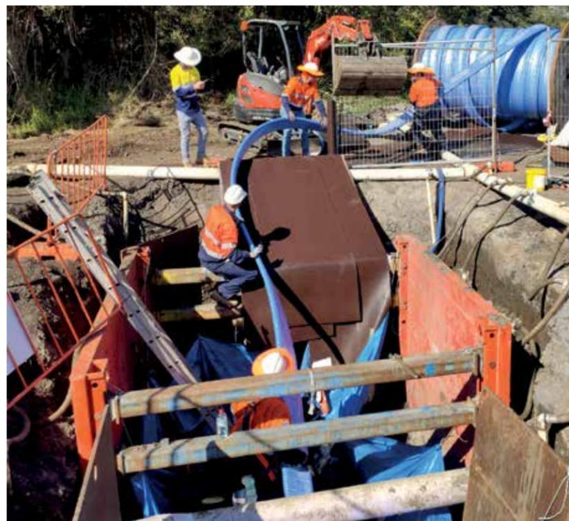
The small installation footprint is small. Installation of 800 metres DN 300 Primus Line in a sewer rising main through an existing maintenance chamber. Primus Line can also be used to renovate vertical pipelines.
