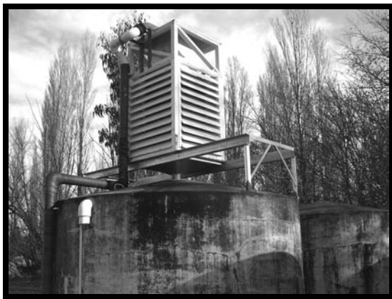
Figure 8: Simple aeration unit
