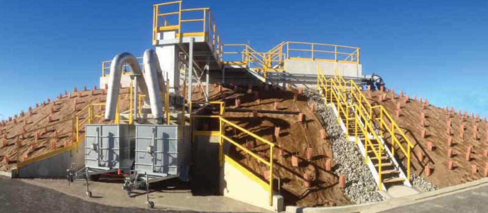
The step screens that form part of the new domestic wastewater treatment plant on Aorangi Road, Seadown, Timaru. In the foreground, the peak flow pump station.
