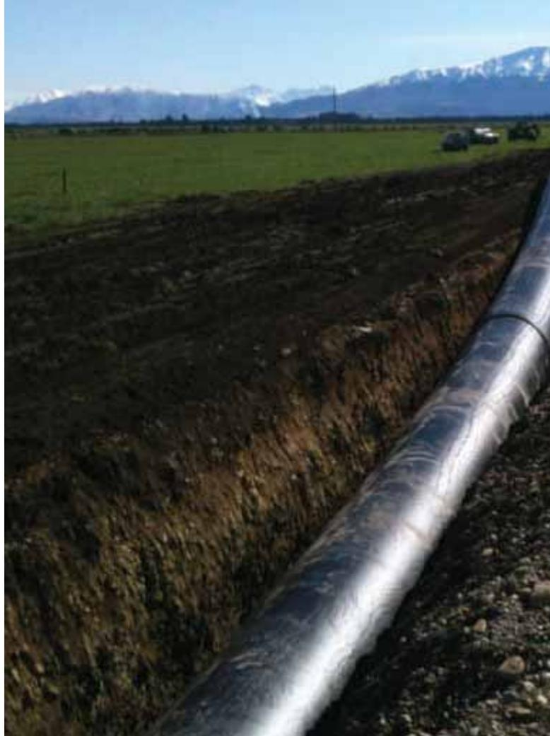
1600mm diameter HDPE pipe being laid across the Canterbury Plains
