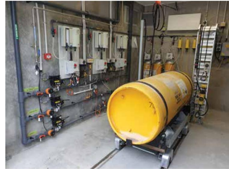
The water is chlorinated prior to being stored in the reservoir above the township. This picture shows the Pahiatua Water Treatment plant chlorine room.
