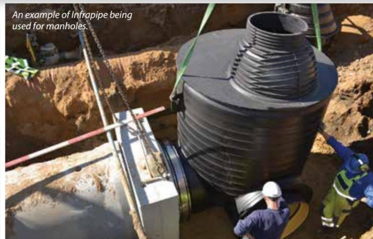
*An example of Infrapipe being used for manholes.*
