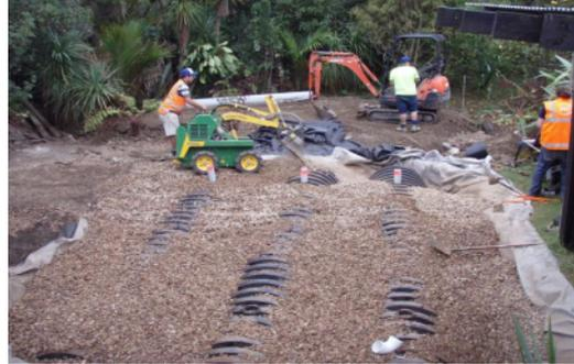
Photographs 5,6,7,8: Construction of MaxxTank
