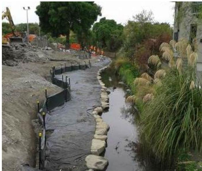
*Photograph 6 & 7: Left: Eel pipes ('tuna townhouses') being installed along the rock edging for Dudley Creek Work Package 1. Right: Eel caves similar to this one along the Avon River also provide cover for larger eels (© EOS Ecology)*
