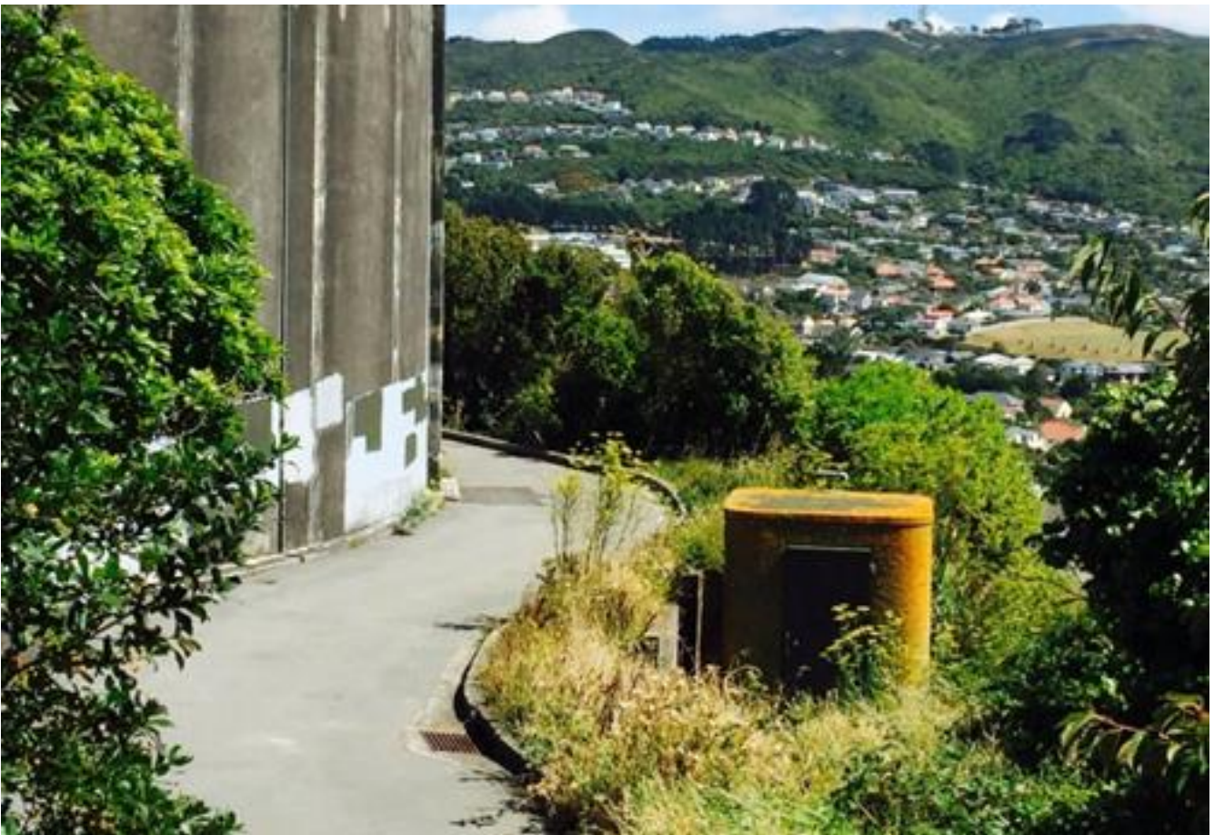
Photograph 4: Typical TDI hut Johnsonville, Wellington
