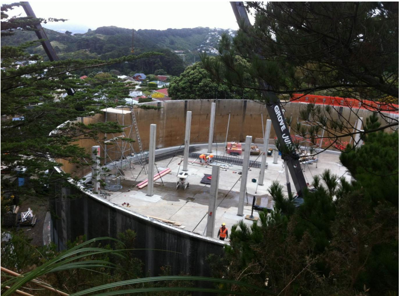
Photograph 1: Seismic upgrade of Carmichael reservoir (7.8ML).
