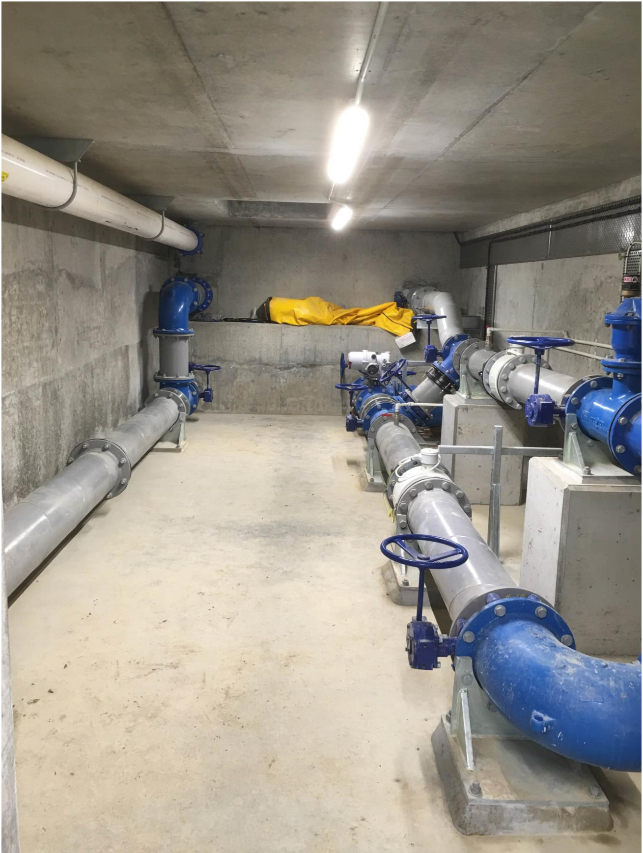
Photograph 3: Melrose reservoir (2.2ML) tunnel (2016)
