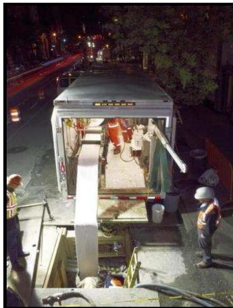
**Figure 15: Insertion of the liner**
