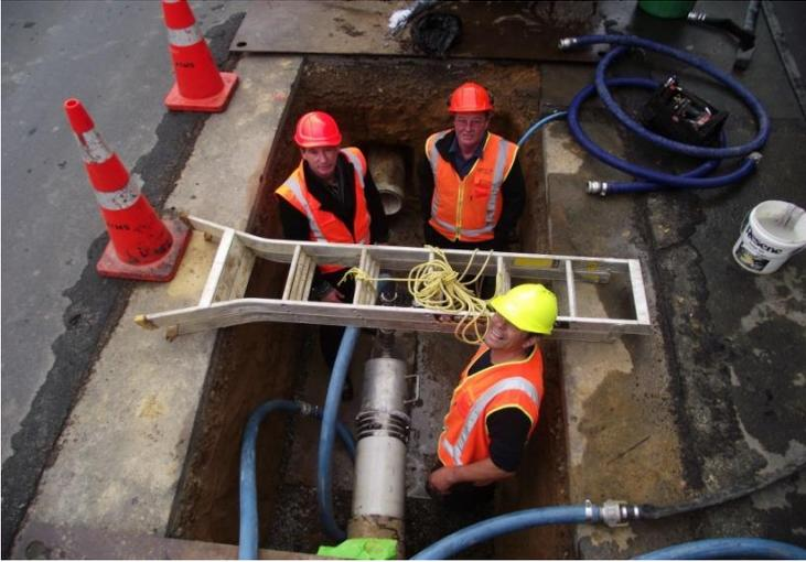
**Relining Pit:** 'Pig Catcher' in action, catching the forming swabs as they are propelled through the line during the forming and curing process
