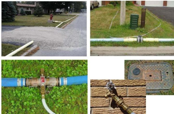
Figure 2: Temporary water supply
