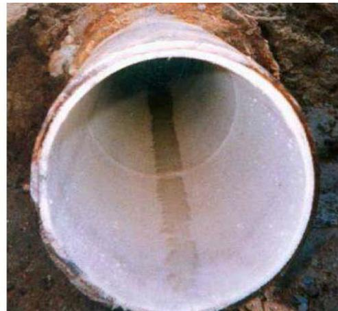
Figure 19: Pipe rehabilitated with AQUA-PIPE®
