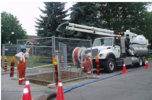
**Figure 6: Trench box and fencing**
