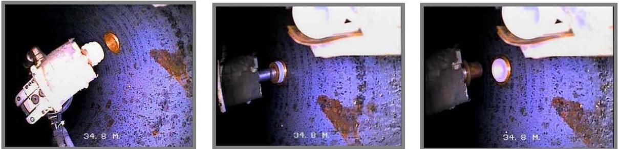
**Figure 12: Plugging service connections**
