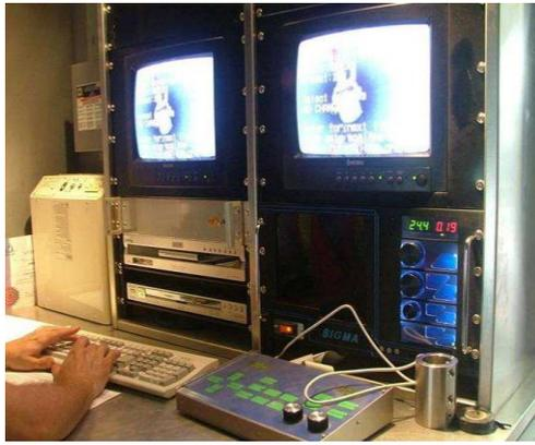
**Figure 11: Control panel for CCTV inspection**
