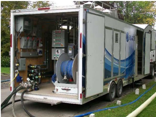
Figure 18: Curing with hot water
