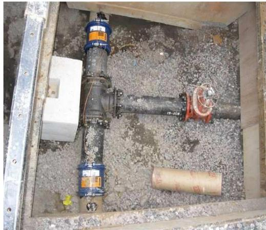
**Figure 22: Typical reconnection in an insertion pit**
