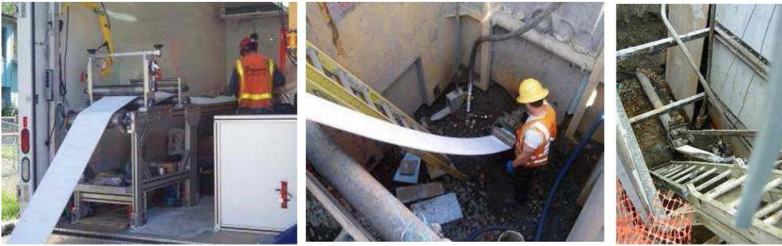
Figure 16: Insertion of the liner
