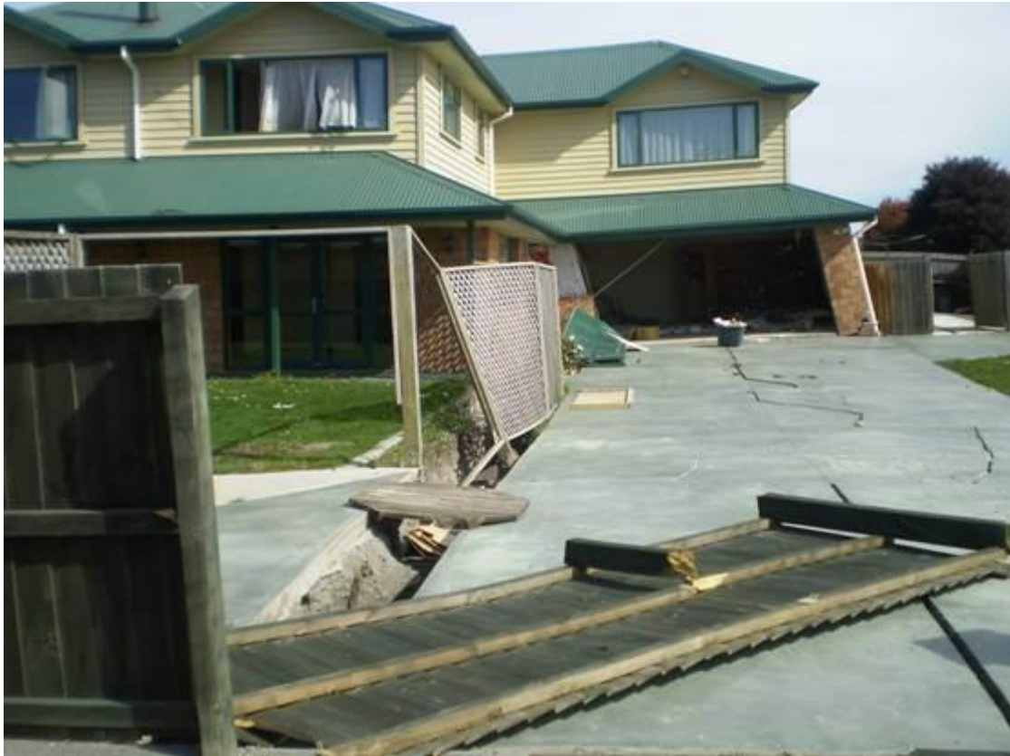
Figure 7. Liquefaction-induced lateral spreading through the foundation of a house after the magnitude 6.3 Christchurch earthquake of 22 February 2011, location unknown.
