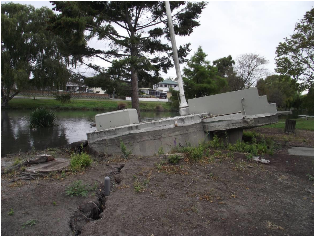
Figure 4: Buoyancy of a pump-station floated up to 500 mm out of the ground by liquefaction adjacent the Avon River near the eastern end of Morris Street, approx. 10 km from the epicentre after the magnitude 6.3 Christchurch earthquake of 22 February 2011. (Photo: D. Beetham, GNS Science)
