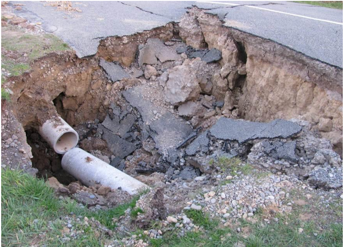
Figure 8. Damage to underground infrastructure from liquefaction, in this case lateral spreading has pulled a pipe joint apart in Cashmere after the magnitude 7.1 Darfield earthquake of 10 September 2010.
