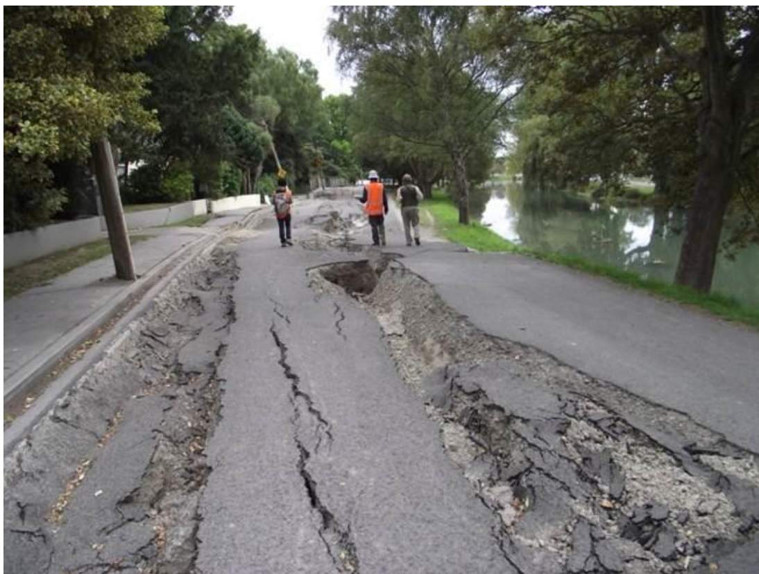
Figure 5: Lateral spreading fissures run parallel to the Avon River in Avonside Drive, Christchurch, approx. 10 km from the epicentre after the magnitude 6.3 Christchurch earthquake of 22 February 2011. (Photo: D. Beetham, GNS Science)
