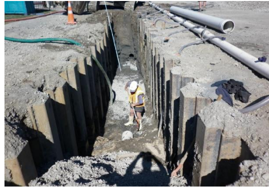
Figure 4-14. Use of sheet piles in pipeline construction
