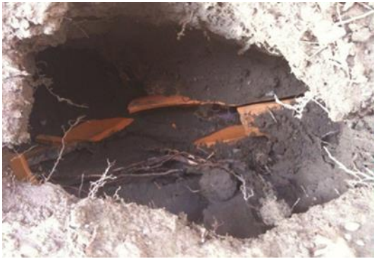
Figure 4-13. Failed earthenware pipe
