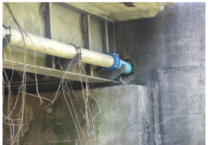
Figure 4-12. Pipe running through concrete abutment of a bridge
