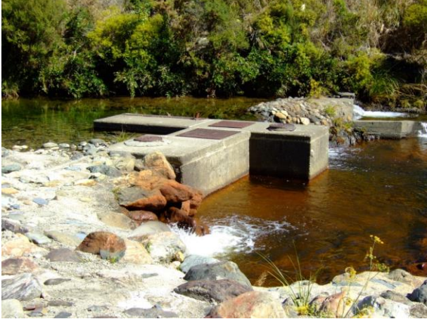
Photograph 5: Intake weir and backfeed discharge, Maitai River
