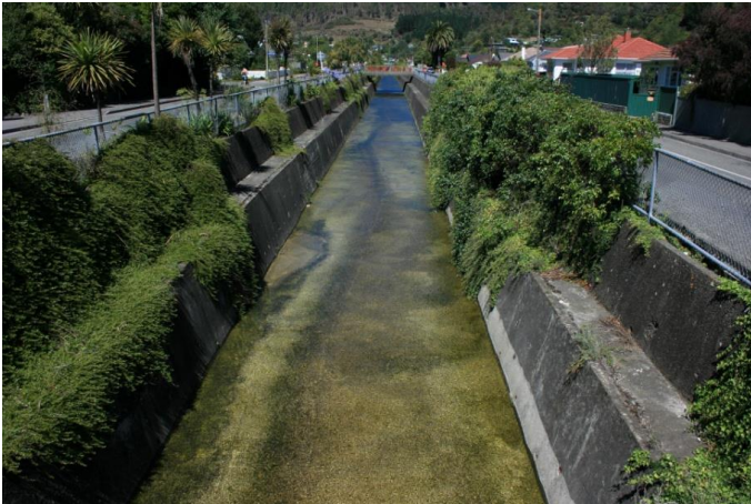
Photograph 6: Brook Stream concrete channel, Nelson
