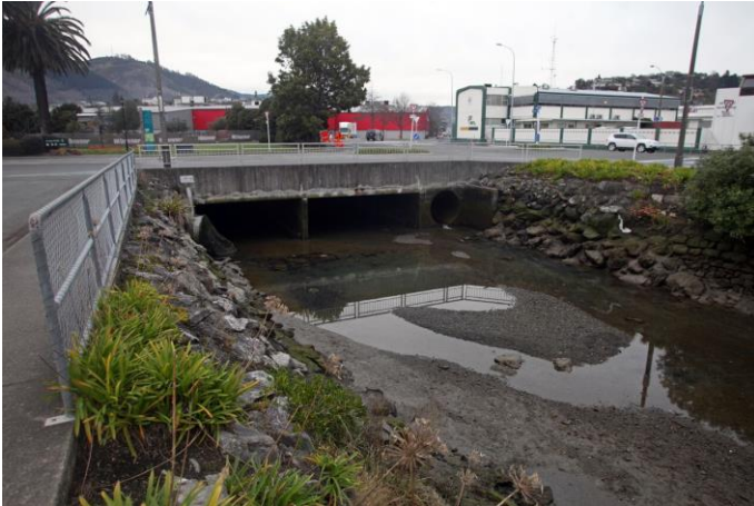
Photograph 7: York Stream culvert, Maitai tributary, Nelson
