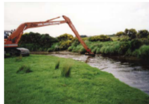
Channel excavation work carried out from the side where the least disturbance will be caused.
