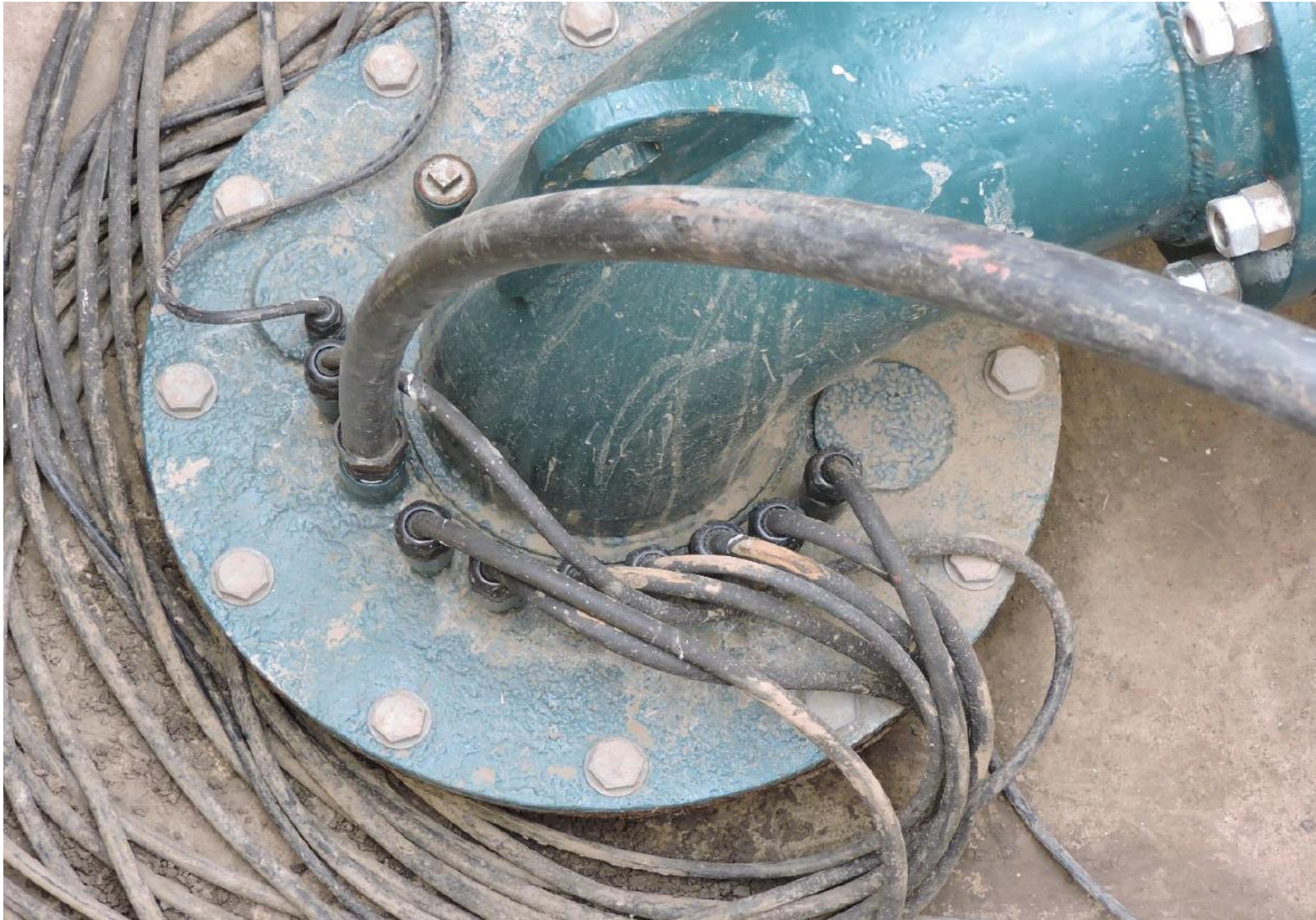
Photograph of Cable Ports
