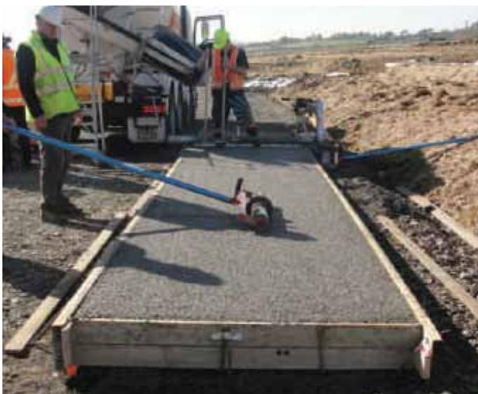
Figure 6 – Advanced porous concrete test panel being poured on-site
