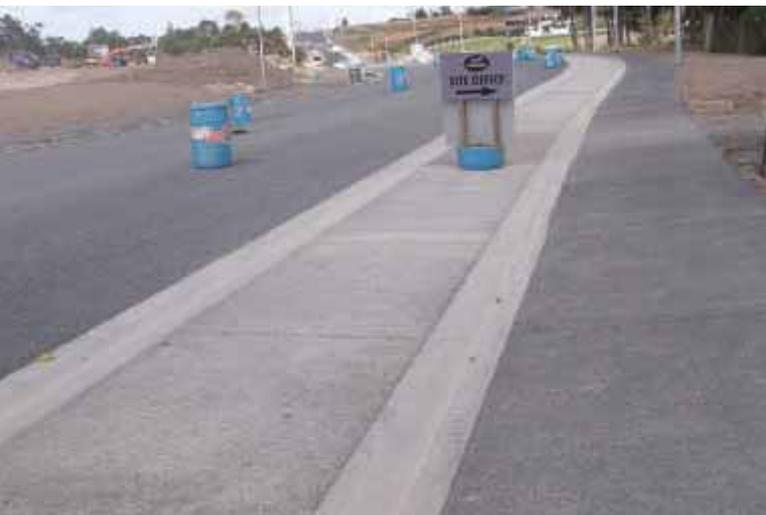
Figure 4 – Porous concrete section at Northside Drive West with v-drain
