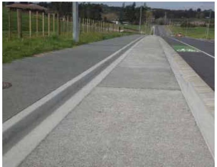
Figure 5 – Porous concrete section on Northside Drive West at 7% longitudinal slope
