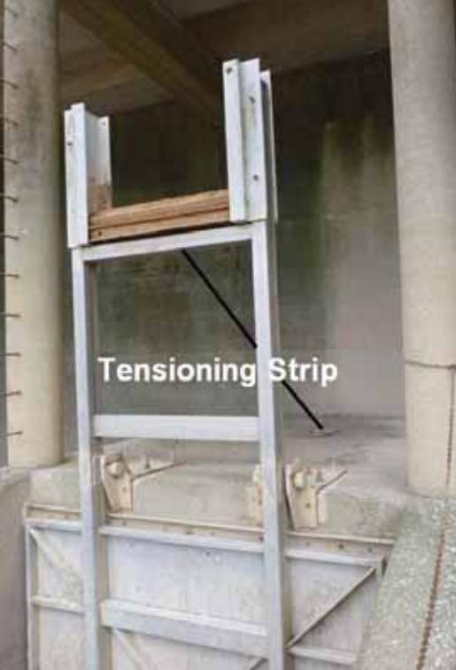
Photo 5 – Tensioning strip to keep gate partially open
