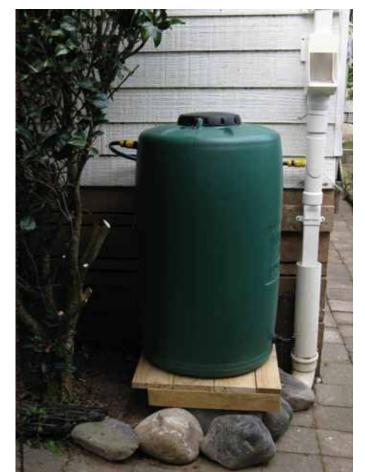
"Roof-collected rainwater can contribute significantly to a sustainable water strategy during disasters like earthquakes, when the lifelines of centralised water infrastructures are compromised. The findings of this pilot study show that rainwater harvesting by the home owners themselves can be a realistic option for a safe water supply, in terms of costs, simplicity of installation and maintenance."
