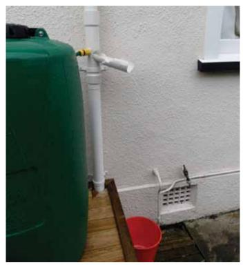
Figure 4 – Full tank and additional water being collected in buckets via diverter chute
