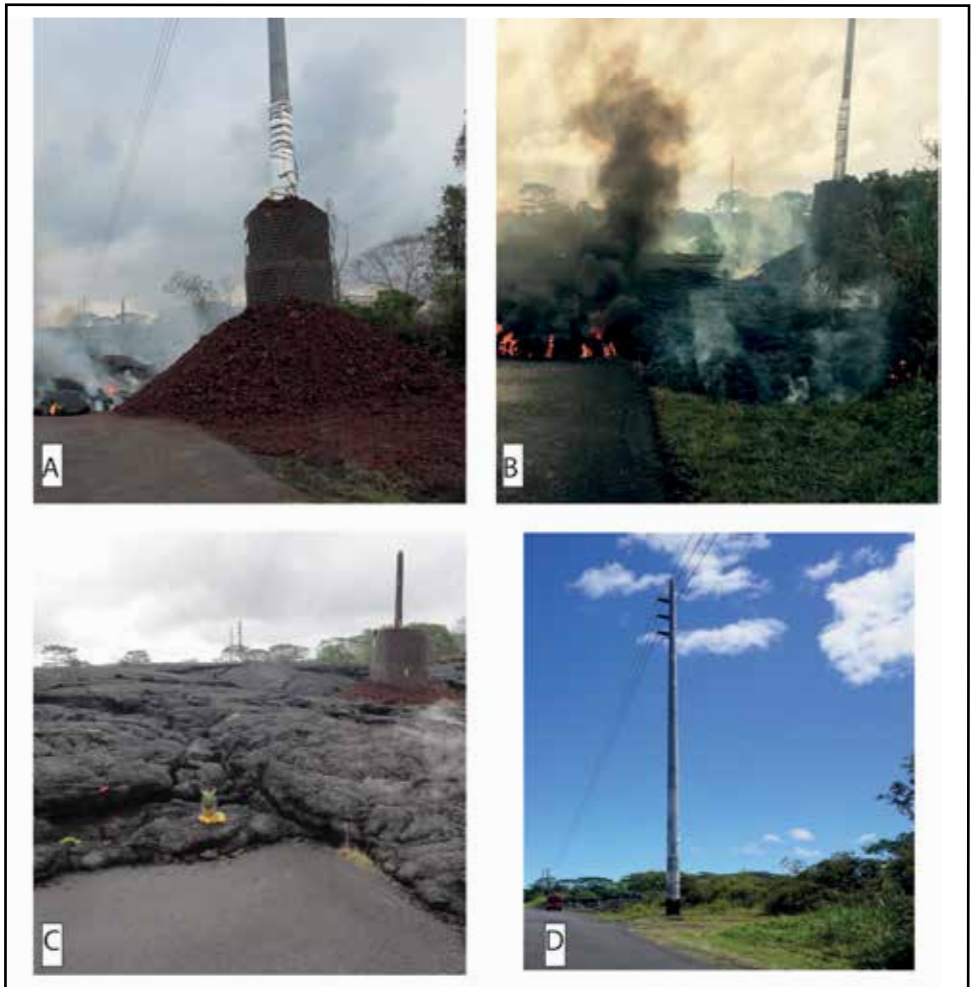
Figure 2: Images of the HELCO power pole protection structure as it was inundated. Image A shows the lava flow approaching the structure. Image B shows the road burning and the lava flow surrounding the structure. By 4 November 2014, the pole had begun burning from below. HELCO disconnected the electric lines and allowed the pole to burn without pulling the electric lines down. Image C shows the remaining pole on 4 November 2014. Image D is from March 2017 and shows the new metal pole that has been installed since the flow ended. Images A through C are courtesy of the U. S. Geological Survey.
