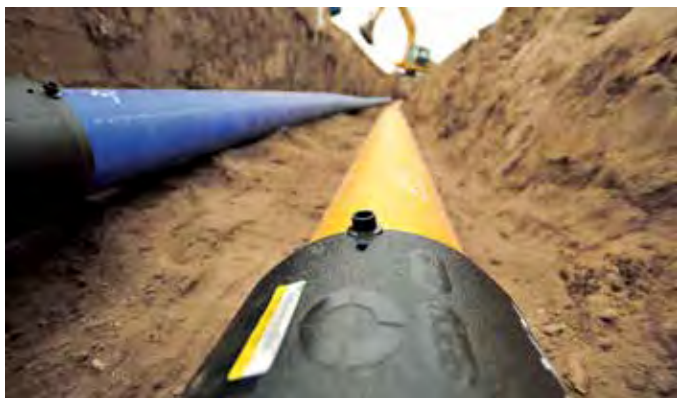
AGRU is always ahead of its time thanks to continuous innovation. Electro-socket fittings proven in millions of applications are manufactured from stress crack resistant PE 100-RC material.
