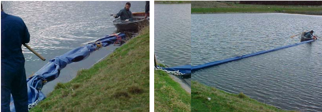
Figure 9-4 Baffle being installed at Ashhurst secondary pond
