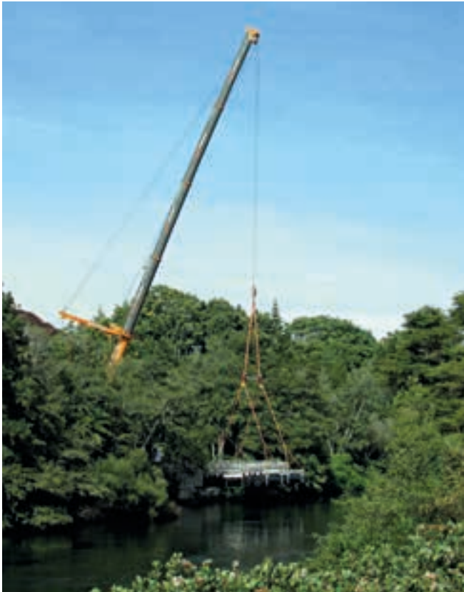
This project involved a floating platform and pump system on the banks of the river that can pump water into the Waikato's intake structure if required when river levels get too low for the existing outlet.
