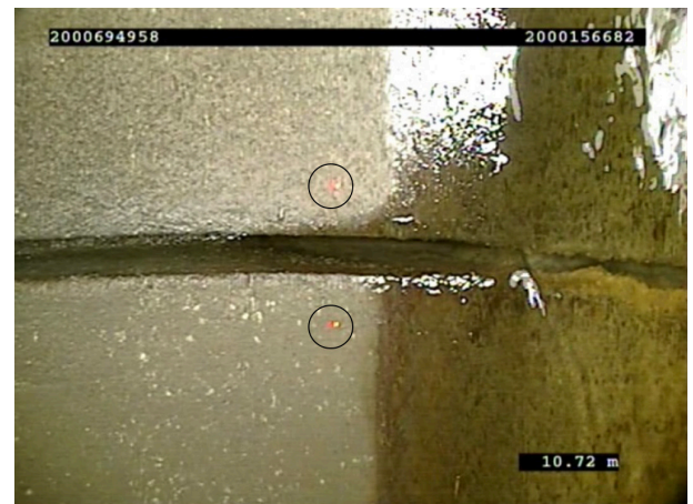
Figure A2.6 – Laser dots projected from the camera head panned towards to pipe wall either side of a joint
