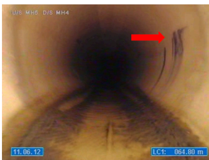
Typical staining from notes written on the liner prior to installation. Staining such as this can also occur where:
