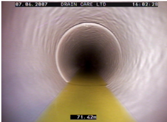
Figure E3.7 – Example of ‘normal’ internal waviness in PVC-U pipe
