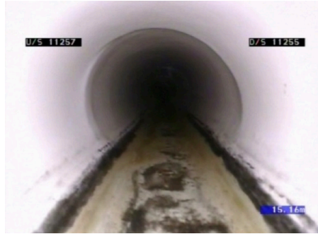
PVC Fold and Form liner installed within a deformed pipe (Ovality >20%)
