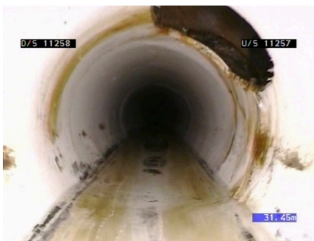
PW1.9.7 – Leak (L)
