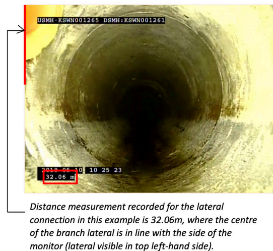
Figure B1.2.13 – Example of measurement to a lateral connection
