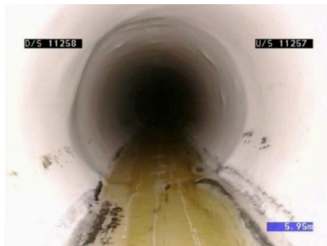
A small displaced and open joint reflected in a Fold and Form liner
