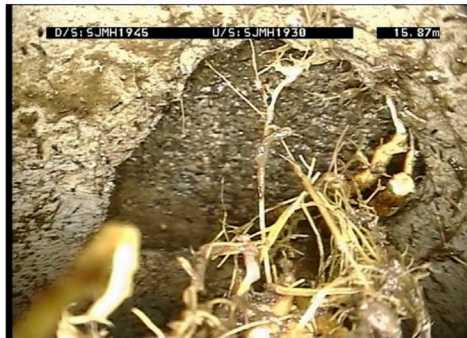
Second photograph taken with the camera tilted and panned towards the defect showing more information that cannot be clearly seen in the first photograph
