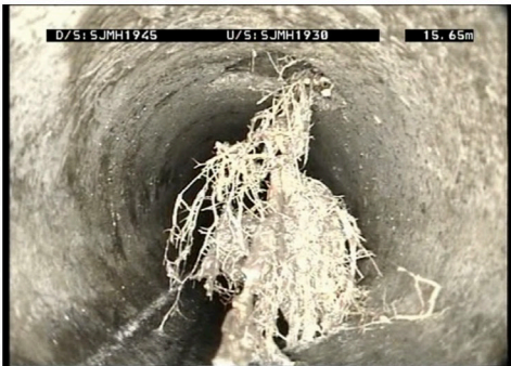
First photograph taken looking 'straight ahead' down the pipe axis, with the camera stopping position as described in clause B1.2.3.3, where the defects (pipe hole and root intrusion) can be clearly seen within the pipe circumference.
