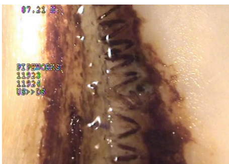
PW1.9.7 – Leak (L)
