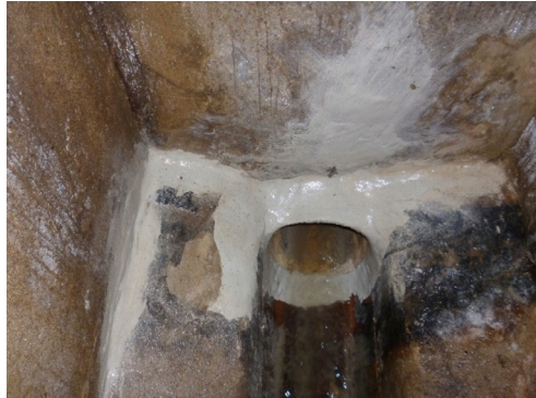
Figure E3.8 – Examples of Liner termination seals (end seals) in manholes
