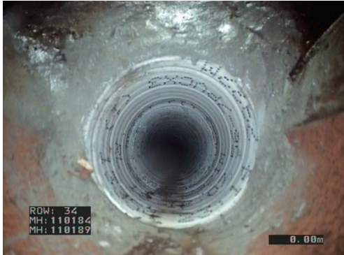
Figure E3.8 – Examples of Liner termination seals (end seals) in manholes
