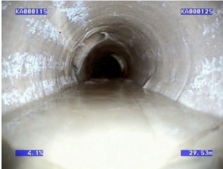
CIPP Lateral Junction Repair, (LJR) installed within a deformed pipe (ovality >20%)
