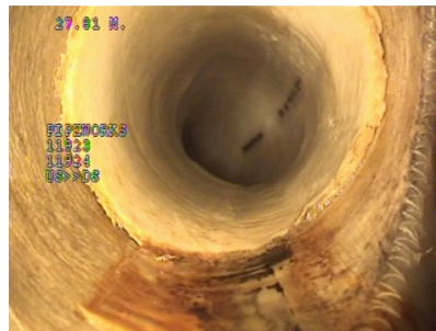
Staining of the LJR invert from flow coming down the lateral. The Lateral has then been lined with a good overlap of lateral liner into LJR. Note the slight discoloration of the resin at the end of the lateral liner.
