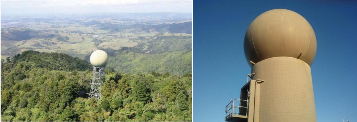
*Photograph 1: The NZ MetService scanning radars at Mount Tamahunga (left, courtesy MetService Ltd.) and Wellington (right)*
