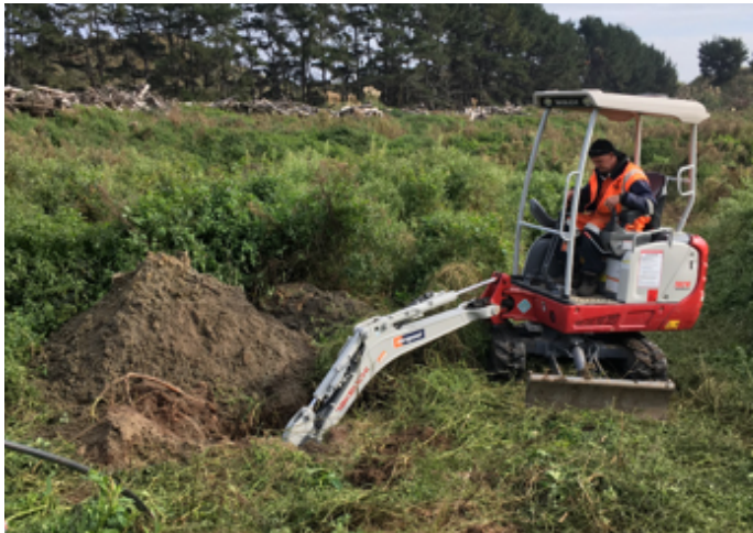
A digger making the 2m deep holes for installing the water flux meters.
