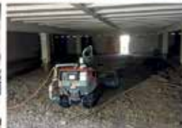
Concrete Treatment’s AQUA CUTTER 410A robot for Hydrodemolition and industrial cleaning.
