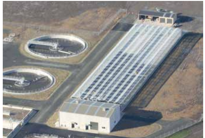
East Selwyn Sewerage Scheme: the solar drying hall.
