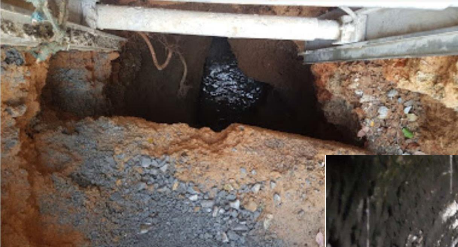
Figure 4 Cavity as first observed, 6 December 2019
