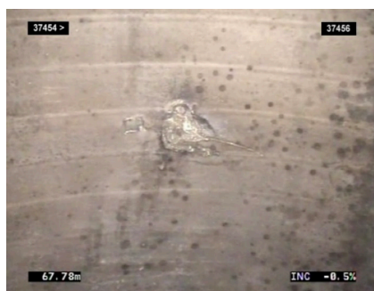
Figure D2 – Examples of vacuum and impregnation patches in CIPP liners
