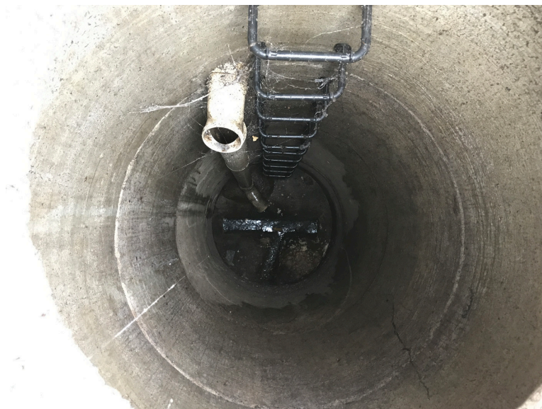
Figure B1.2.4 – Example of view looking down a manhole when the camera (pan and tilt or fixed head) cannot start in the manhole
