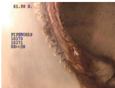
Edge dry, staining present within 'flow zone' of the lateral.
