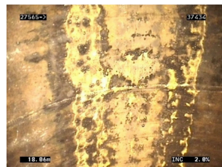
Photo, above, typical staining on the soffit (roof) of a liner, from the lubricants used during installation.
