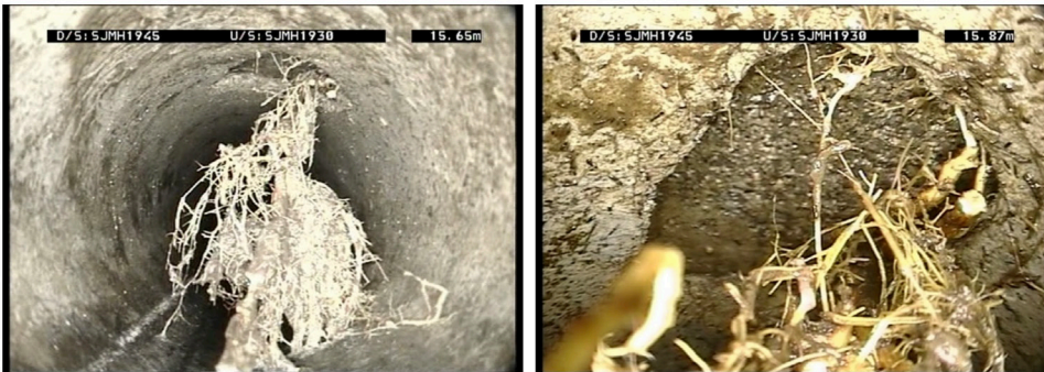
Figure B1.14 – Example of first photograph and second/subsequent photograph showing defect detail without over zooming
