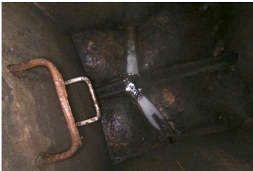
Example 1 st photo showing corroded step rung
