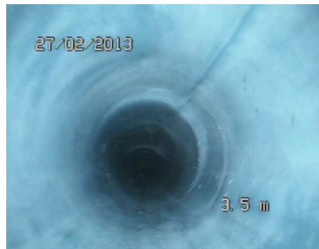
CIPP liner reflecting a joint in an EW pipe
