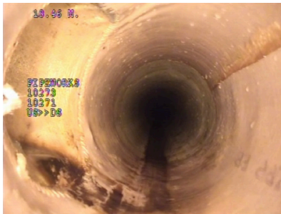
Resin discoloration at the start of an LJR
