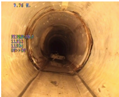
Resin discoloration at the start of an LJR
