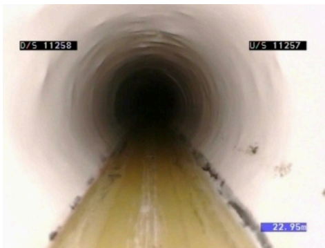
Mirrored irregular shape of the broken existing pipe beneath a Fold and Form liner
