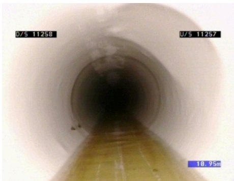
A 'dimple' produced in a PVC fold and Form liner over a lateral connection
