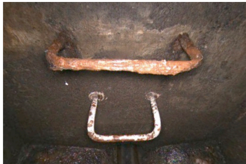
Example 2 nd photo providing a panned view of corroded step rung
