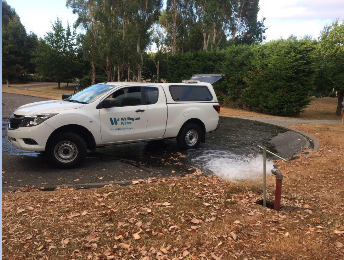
Flushing of the Network
