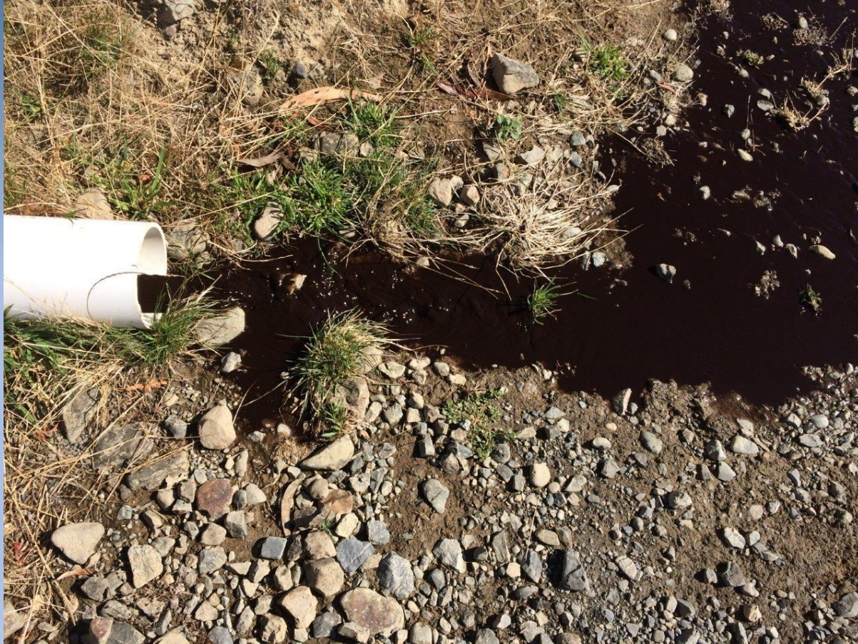
Draining of reservoirs showing manganese deposits and Reservoir Cleaning
