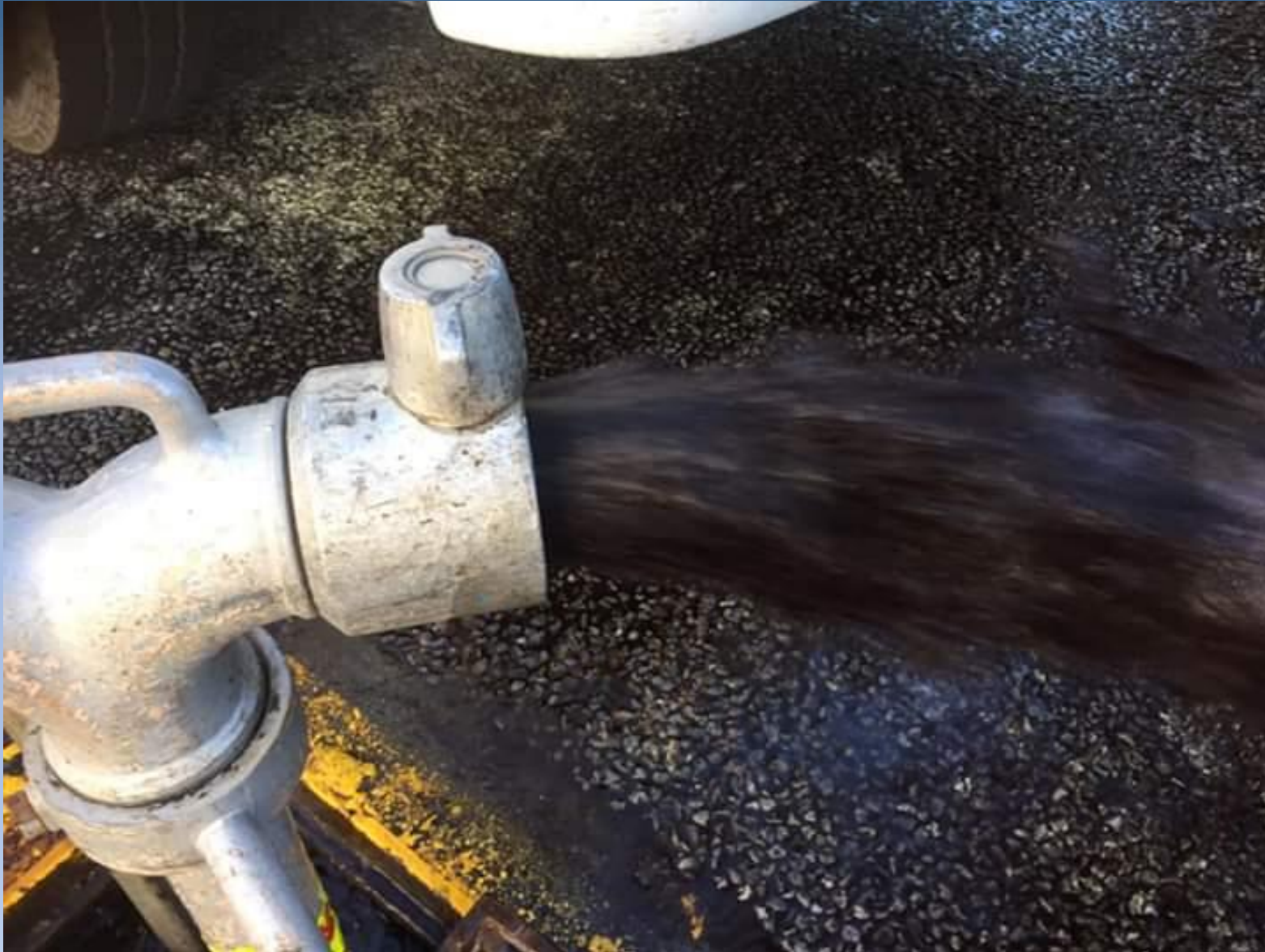
Flushing of agitated manganese due to air-scouring of network
