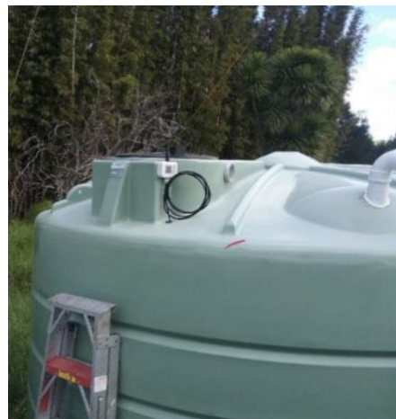
Figure 9.2: Coiling and tying of excess sensor cable.
