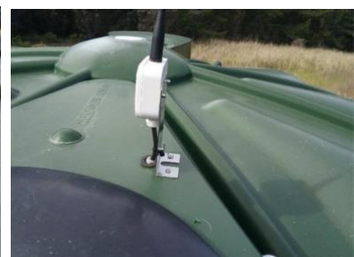
Figure 8.3: Installation of monitor on a plastic tank.
