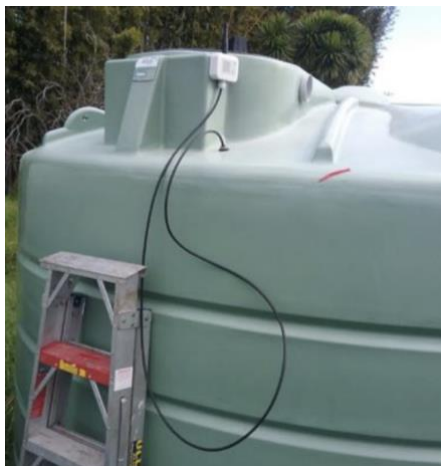
Figure 9.1: Excess sensor cable on tank.
