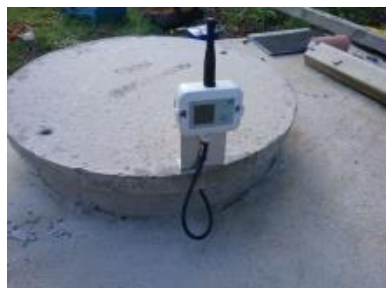
Figure 8.2: Installation of monitor on a new concrete tank.
