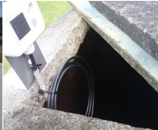
Figure 10.2: Coiling and tying of excess sensor cable inside a concrete tank.
