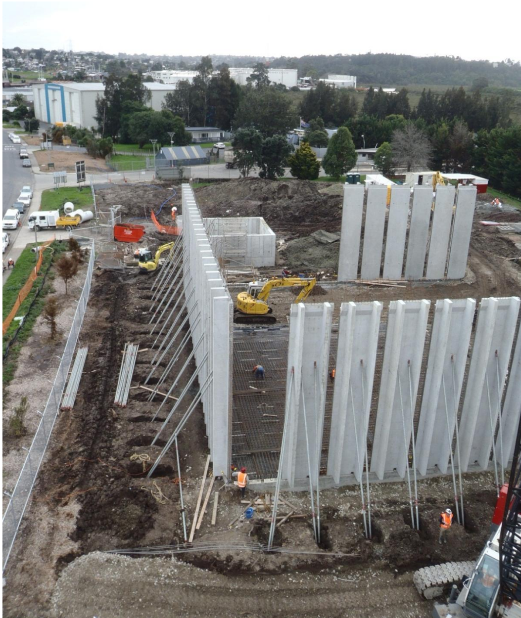
Photograph showing double-tee precast panels partially erected
