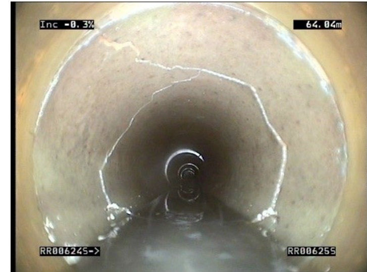
Multiple Cracks (Displaced)
