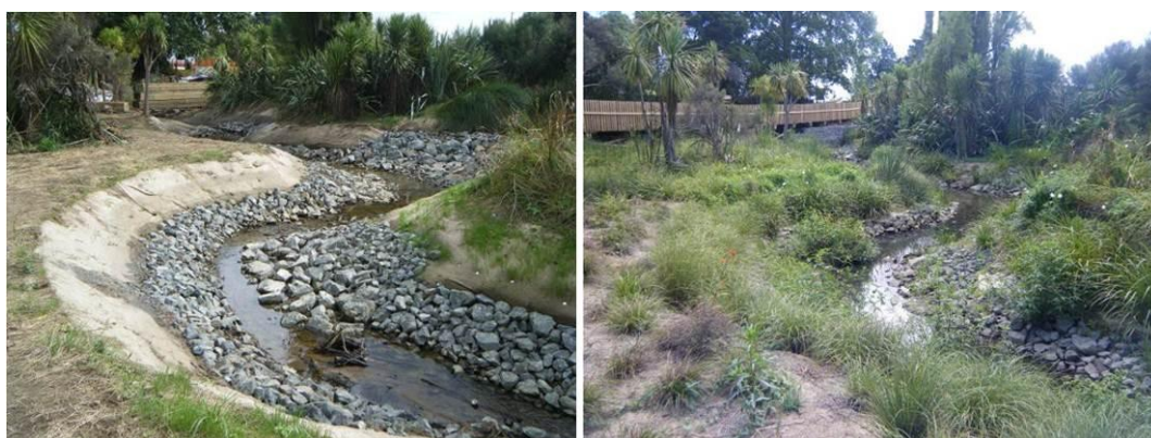
Figure 9: Showing bank and bed modifications through pool and run sequences
