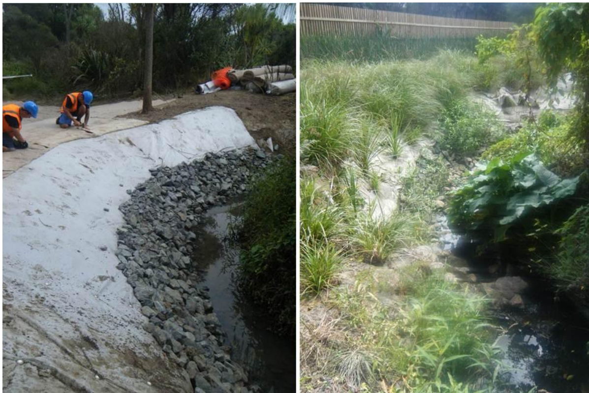
Figure 8: Showing toe armoring and planting after 6 months
