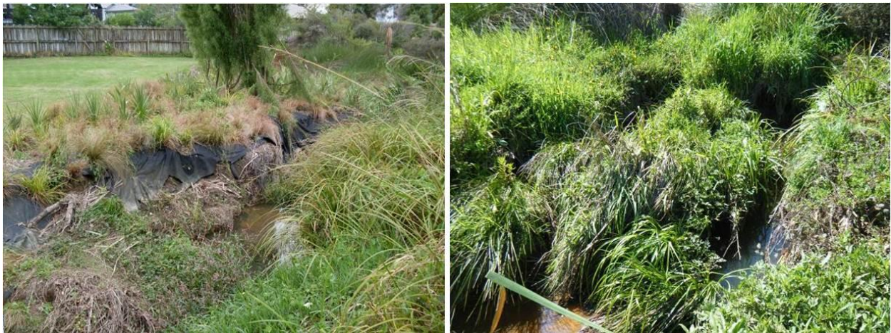
Figure 5: Showing previous attempts to arrest bank slumping and the reduction in channel cross-sectional area
