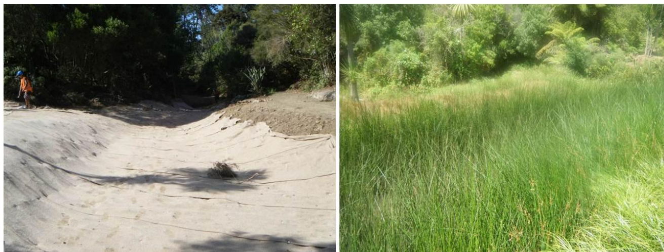
Figure 16: Improved conveyance channel and constructed depression wetland
