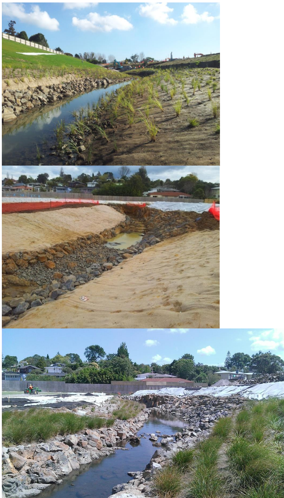
Photo 6 Stream realignment and restoration as part of SH20 works showing early stages of riparian planting and rock riffle pool runs with basalt outcrop retained.
