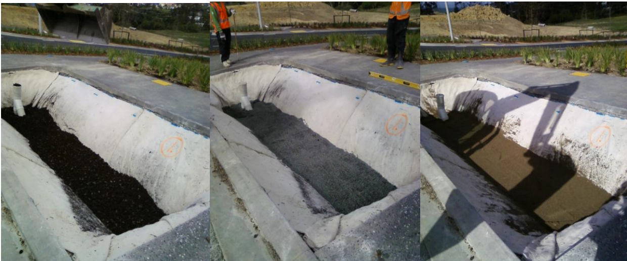
Photograph 2: Rain garden Construction
