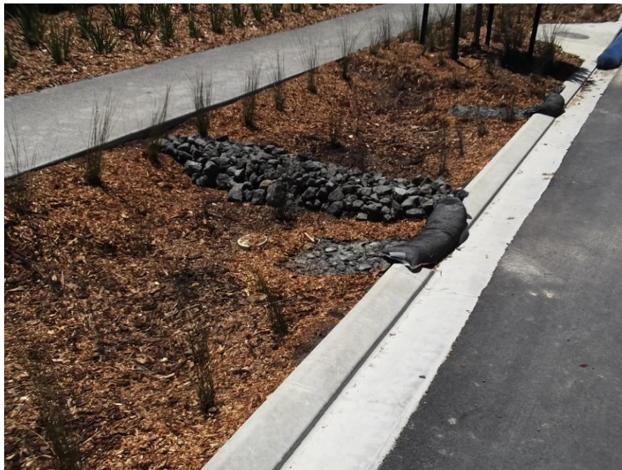
Photograph 1: Constructed Rain Garden
