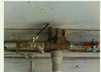
This one is un-testable because it is almost touching the ceiling. No room for test nipples let alone test gauge hoses. Attached to this illegal installation were the test results for this RPZ as follows:
