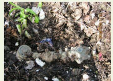
This RPZ had to be dug up before we could find the top of it. No 300mm clearance from the relief valve, the relief is still underground. This installation includes the meter, then a double check, then an RPZ all in one line.
