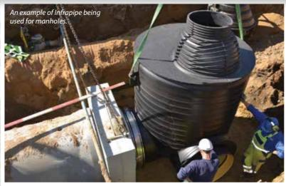
one of the safest forms of plastic. It is solvent resistant and has high strength characteristics. It's the perfect material for pipes and one of the easiest plastics to recycle – it will last for 100 years, then you can dig it up, chip it and use it to manufacture something else.
