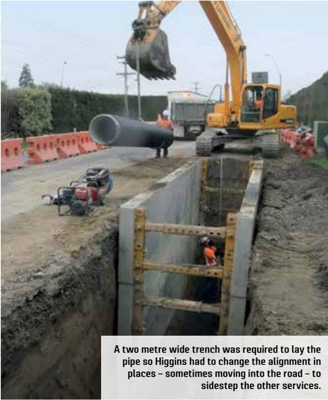
A two metre wide trench was required to lay the pipe so Higgins had to change the alignment in places – sometimes moving into the road – to sidestep the other services.
