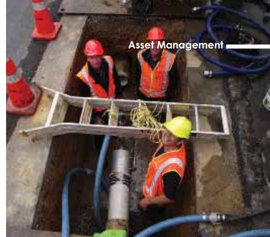
Formed liner is the white extending out of the old AC pipe.
