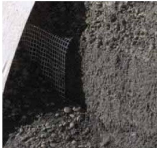
Far left – Geogrid embedment wrapping, Left – Installation of pipes for testing
