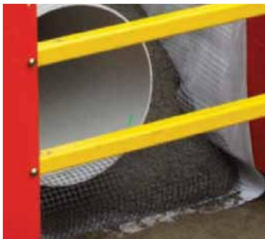
Far left – Geotextile sock over coupler, Left – Embedment installation
