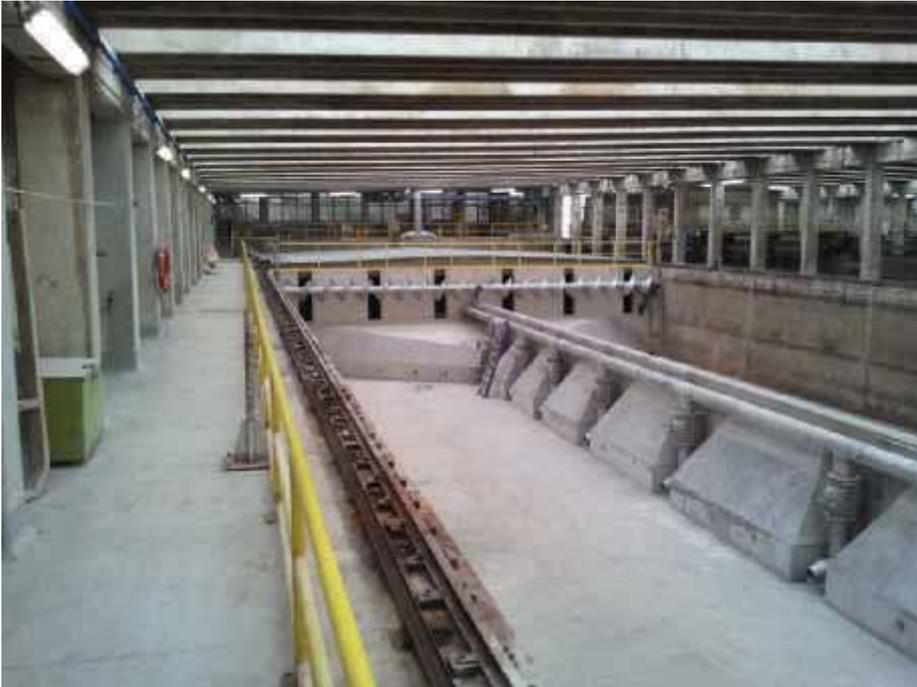
Photograph 1 – Looking to the inlet end of the empty HRAS tank showing the scum removal screw, closer spaced sludge removal ports and covered aeration tank in the background
