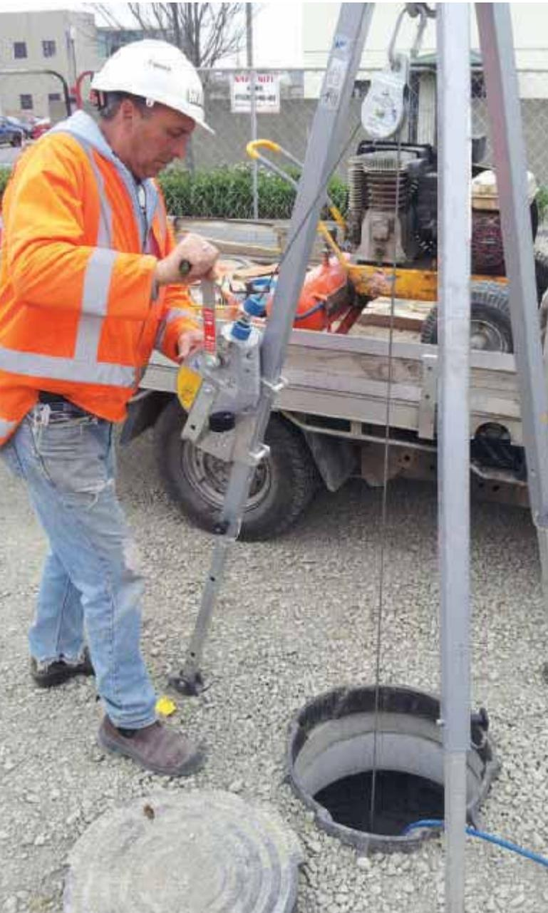
March Construction crew block and test a 50 metre line to locate a leak
