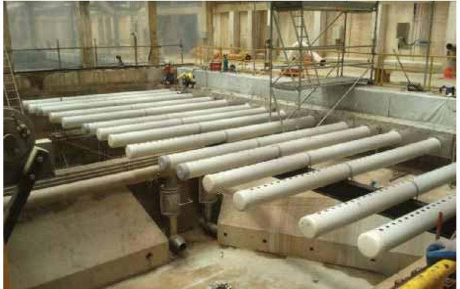
Photograph 4 – Outlet end of HRAS tank during construction, showing the submerged outlet launder tubes
