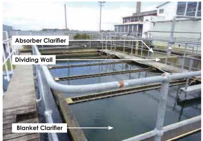
To ensure the plant could continue to treat water during the upgrade, the blanket clarifier was decommissioned and upgraded first, leaving the absorber clarifier to take the full plant flow. The upgrade involved removing all the internals and pouring a concrete base in the bottom of the 'V' of the clarifier (see photo below). A sludge scraper was then installed to scrape the sludge to the inlet end of the clarifier.
