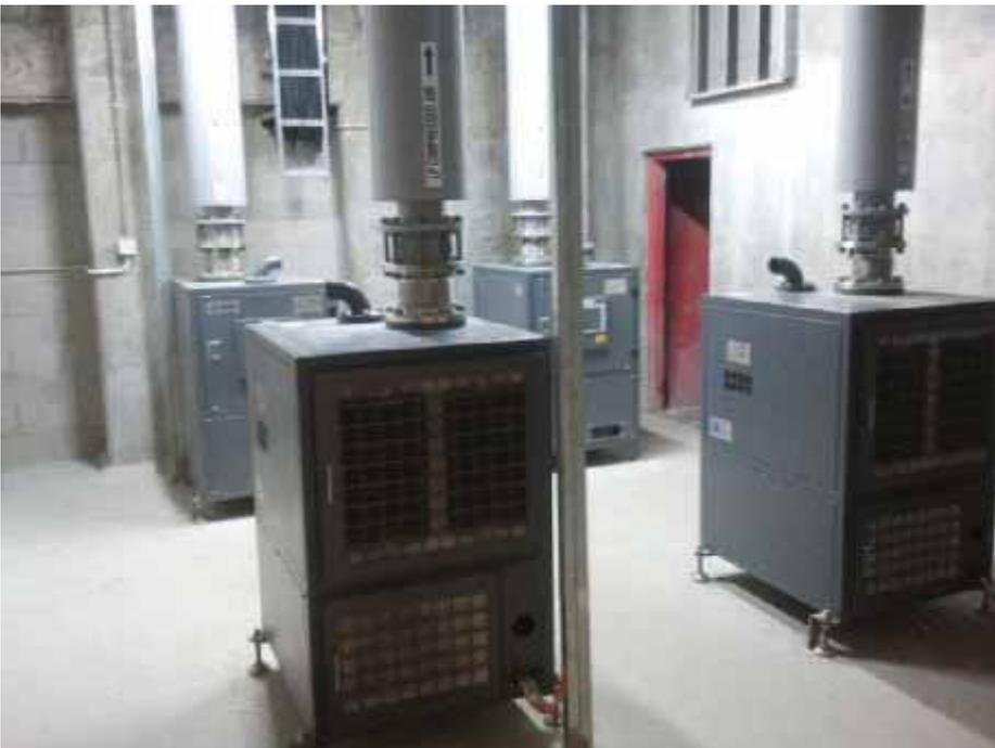
Photograph 2 – K-Turbo High Speed blowers at Tahuna WWTP
