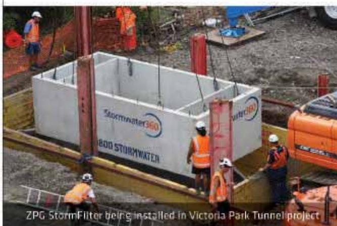
ZPG StormFilter being installed in Victoria Park Tunnel project
