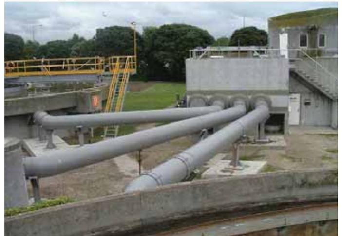
Figure 2 – New pipework to feed the primary settling tanks, and removing plant bottle-necks has increased hydraulic capacity
