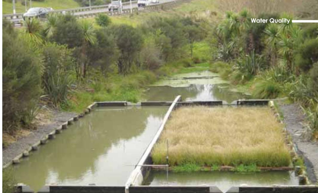
Top left – SH1 to SH16 Link – 2008 Milk Powder Spill, Above left – SH16 Causeway 23rd January 2011 – 6 tonnes of coastal debris cleared following morning tide (Photo courtesy of Peter Mitchell), Above right – SH1 Bifurcated Stormwater Pond – Silverdale Floating Vegetated Island Trial
