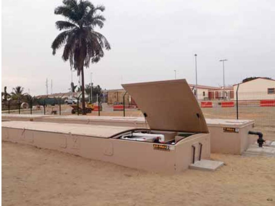
Above – Treatment units installed below ground for reduced visual impact, Right – Control panel installed in secure onsite service building
