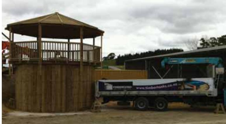
A different approach to utilising a rainwater harvesting tank at the Kerikeri Riding School. A viewing platform/gazebo has been erected overlooking the equestrian dressage arena on the newly constructed 45m<sup>3</sup> Timbertank. Water is collected from the roof of the adjacent indoor arena and piped to the tank.
