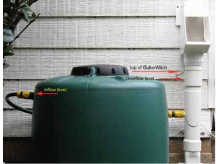
Figure 3 – Correct arrangement of diverter and inflow and outflow pipes
