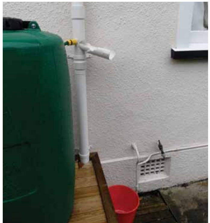
Figure 4 – Full tank and additional water being collected in buckets via diverter chute
