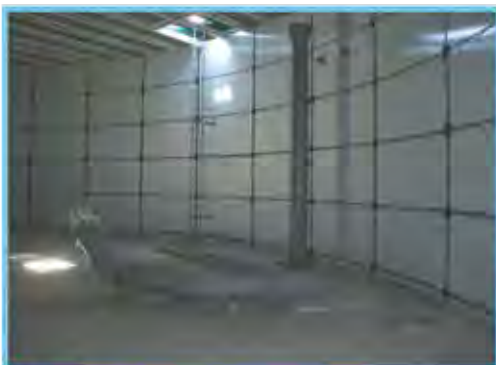
Photo 1: Fusion Bonded Epoxy internal tank coating (no liner!)
