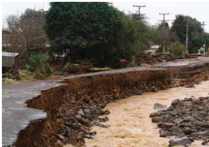
Figure 1 – Damage to Te Puru Creek Road after the "Weather Bomb 2002"
