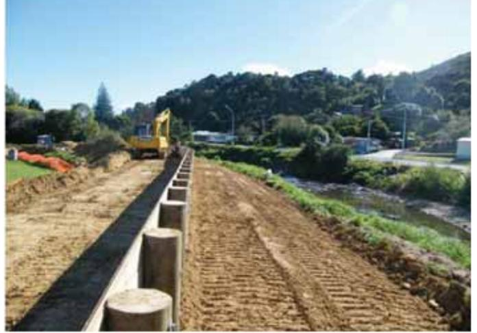
Figure 4 – Flood wall construction
